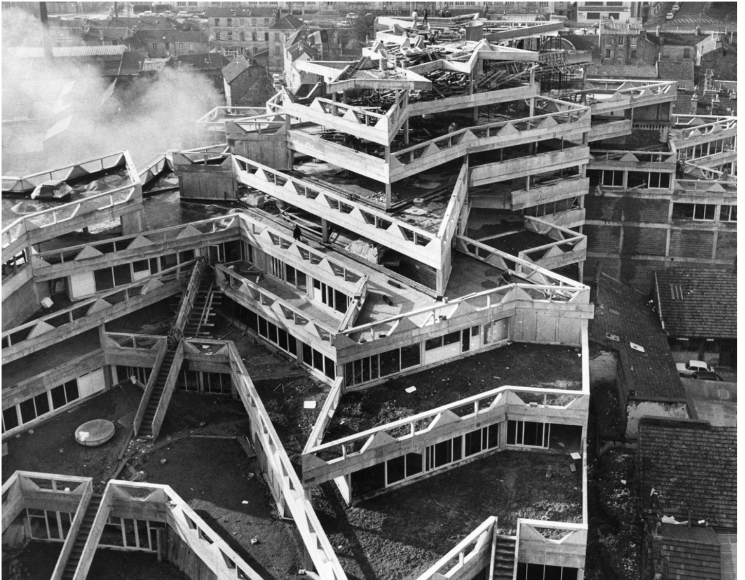
2.8 Jeanne Hachette 'tranche 1' during construction (1973)
